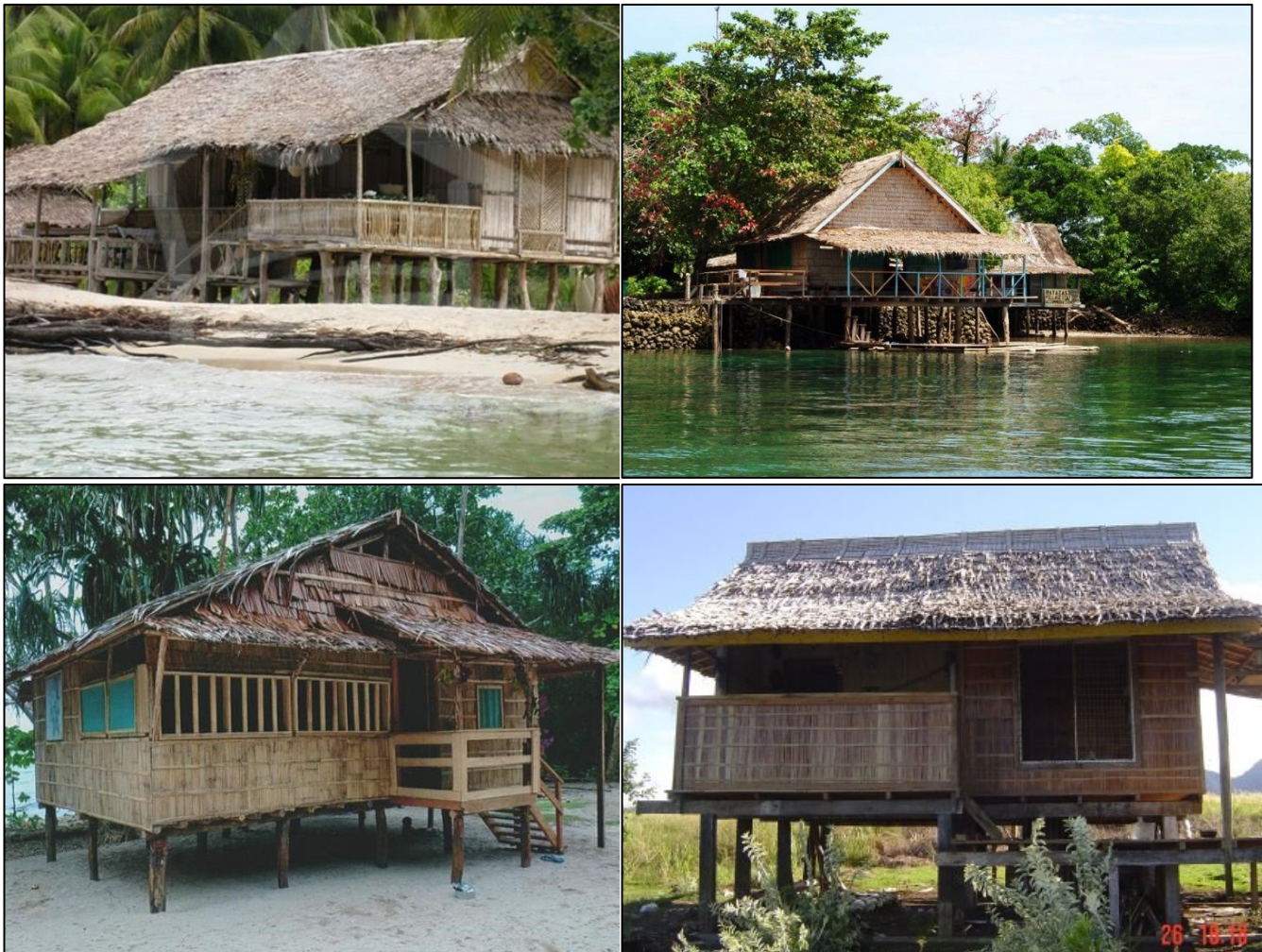
Empty tourist bungalows: "If you build it, they will come" is a sad untruth for many village tourism hopefuls
